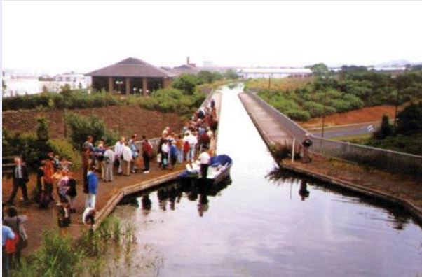
Fig. 7: The Scott Russell Aqueduct on the Union Canal near Heriot-Watt University, 12 July 1995. For the technically minded, the aqueduct is 89.3 m long, 4.13m wide, and 1.52m deep.
